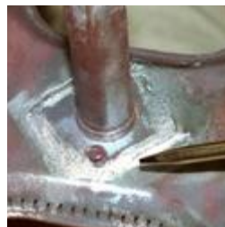
Pyro-Putty® 653 seals corroded burner manifold.
