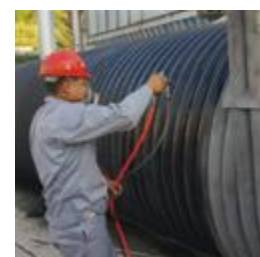
HiE-Coat™ 840-M coats industrial heat exchanger.
